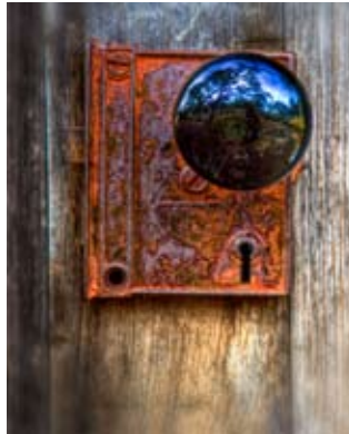
7. Detail of Historic Building by Rose Epps
