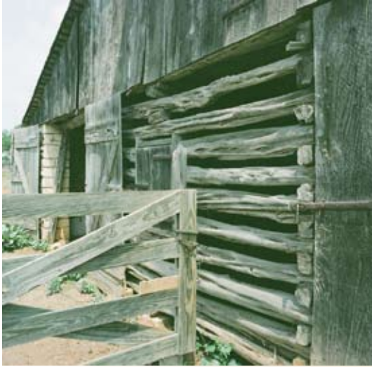
Old Barn original shot
